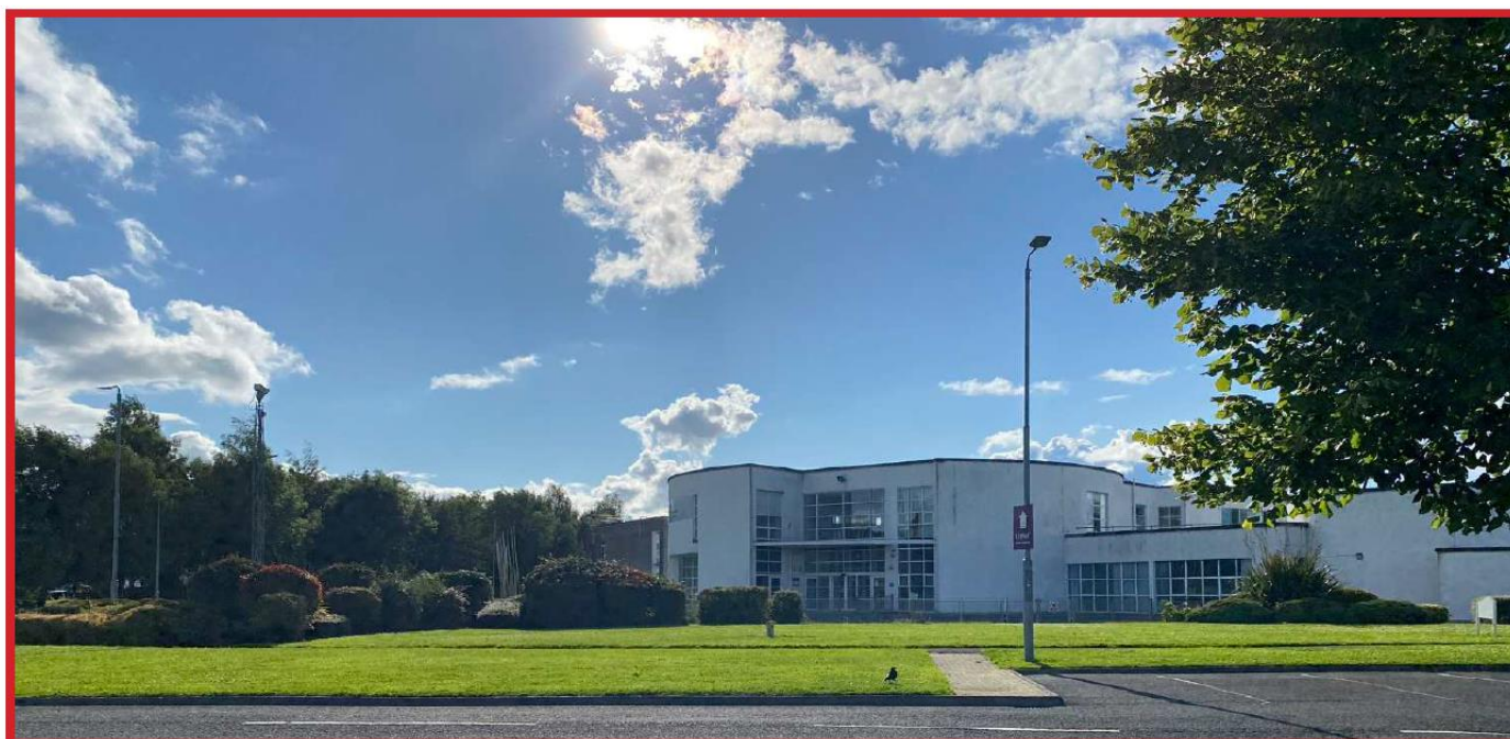
Above: Under the proposal for Thurles Connected Campus, over 2,000 FET and HE places will be provided in the existing TUS facility on Racecourse Road in Thurles
